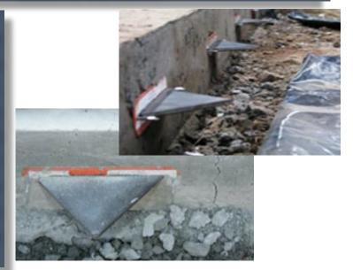
All top commercial designers are designing slabs with ACI 360R-10 - Guide to Designs of Slabs-on-Ground. They make it clear the tapered plate dowel
